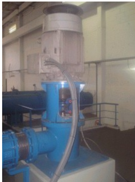
Figura 137-Electrobomba (C.A.S).
